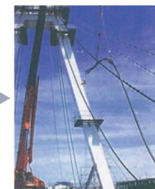
3 | Drawing & fixing of dead anchor
