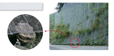
It is not desirable that important facilities built to prevent rockfall accidents loose their function in short times due to corrosive deterioration of any particular component member. Based on this idea, standard plating specifications assure at least 50 years of corrosion resistance in mountainous areas, which are typical locations for such facilities.
