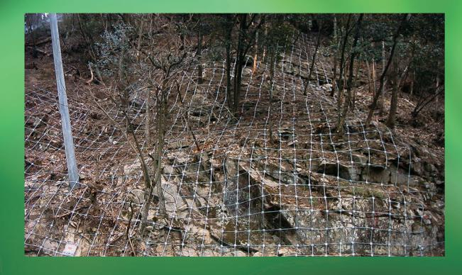
Rope Net that helps eliminate the rockfalls, also protects environment. If you use Rope Net with a net or other systems that prevent rockfalls not only relatively large rocks, but also of small stones.
