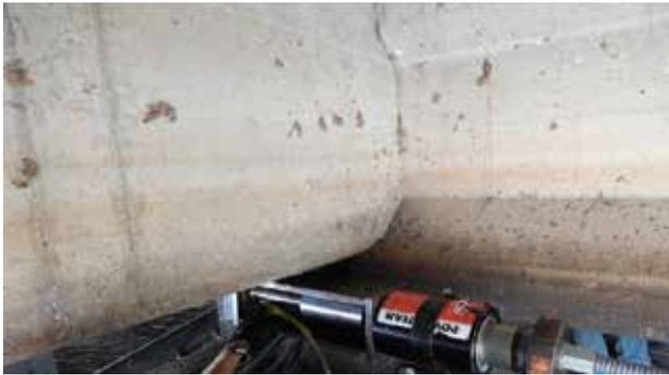
Post-tensioning cable with load cell
