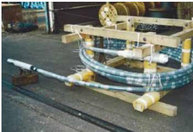
Fig. 2—Post-tensioning 40 mm (1.57 in.) diameter CFCC with pre-installed anchoring devices on both ends.
