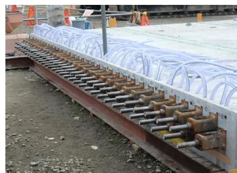
Photo-3 Terminal of Post-tensioning (Cut after grout strength development)
