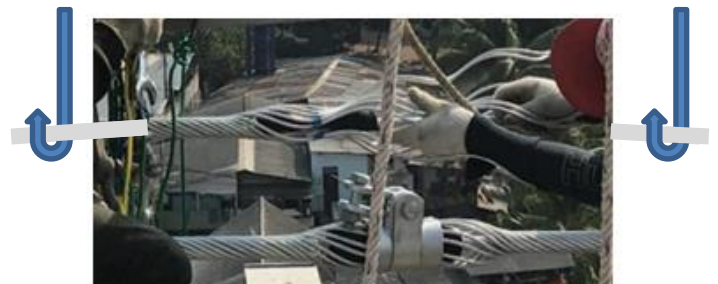
Installation of Armor rod and suspension clamp
