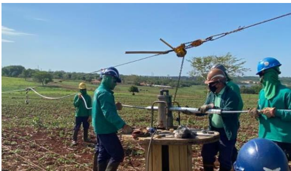
Installation of midspan joint on the ground
