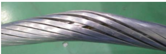
Strand opening due to sharp "local" overbending
