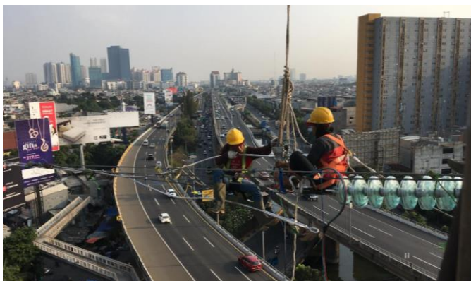
Installation of Deadend clamp on the tower
